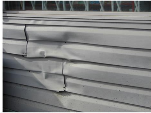
Vinyl siding will melt if your hot BBQ is too close. No protection from forest fires.
