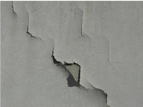
This acrylic stucco was applied without rainscreen to a surface that was not stable.
