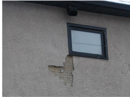
Quality control is difficult with stucco. Poor curing conditions on hot days.
